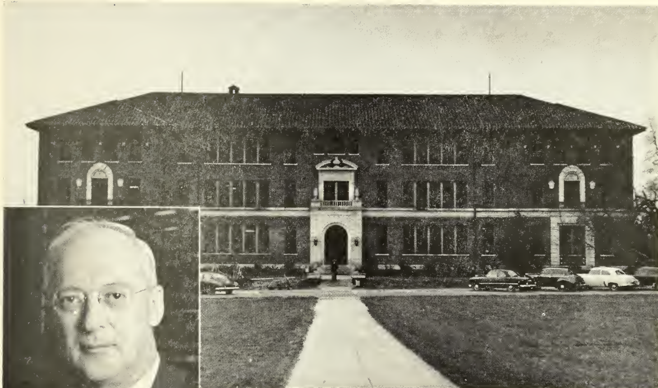
RIGGS HALL — ENGINEERING BUILDING
